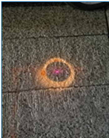
Figure 5. Pavement Marking with Chalk Source: NYCDOT
